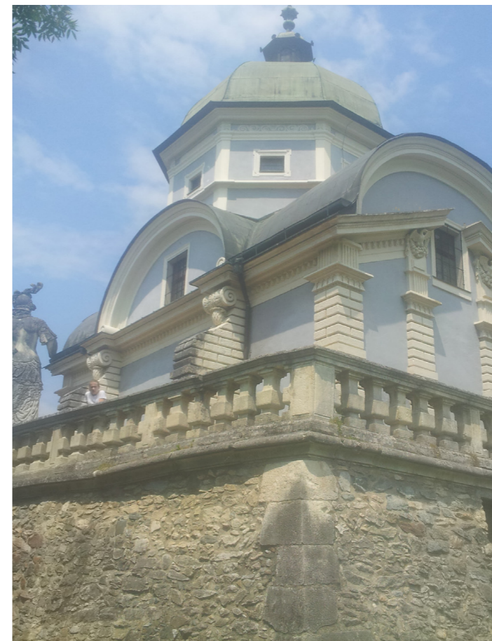
Approached by a steep winding path and steps, one emerges below the platform on which it sits
