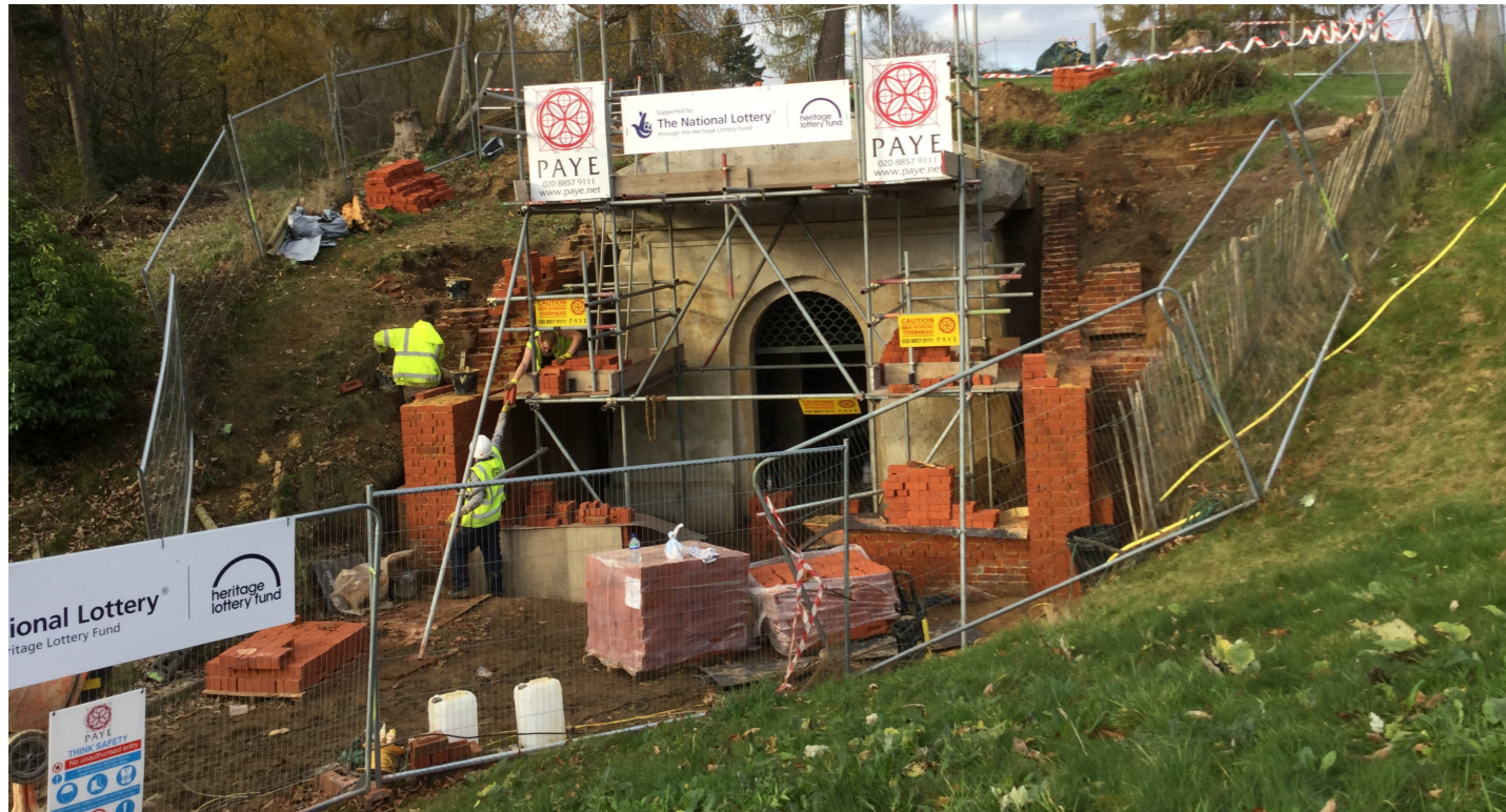
External courtyard walls being rebuilt ready for rendering
