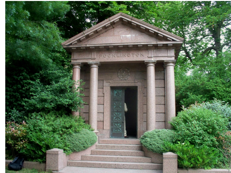
Pocklington Mausoleum - Front Facade
