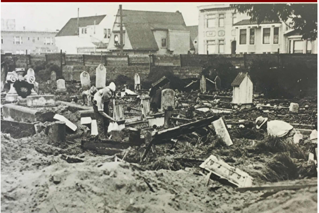
Disinterment work in Odd Fellows Cemetery, San Francisco. Many bodies were missed during these cemetery removals and remains are still found during excavations for new buildings on former cemetery sites. Monuments were broken up, dumped in the Bay, or used in public realm works.
