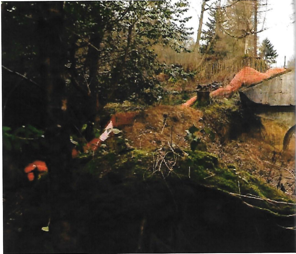
Hope Mausoleum after partial uncovering in February 2010
