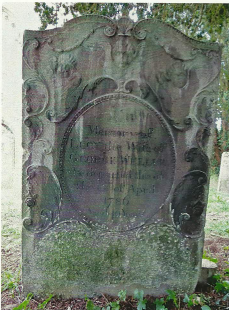
The Weller headstone in 2012. Soot is eroding the surface of the Portland stone, and the clarity of inscription is in sharp decline.
