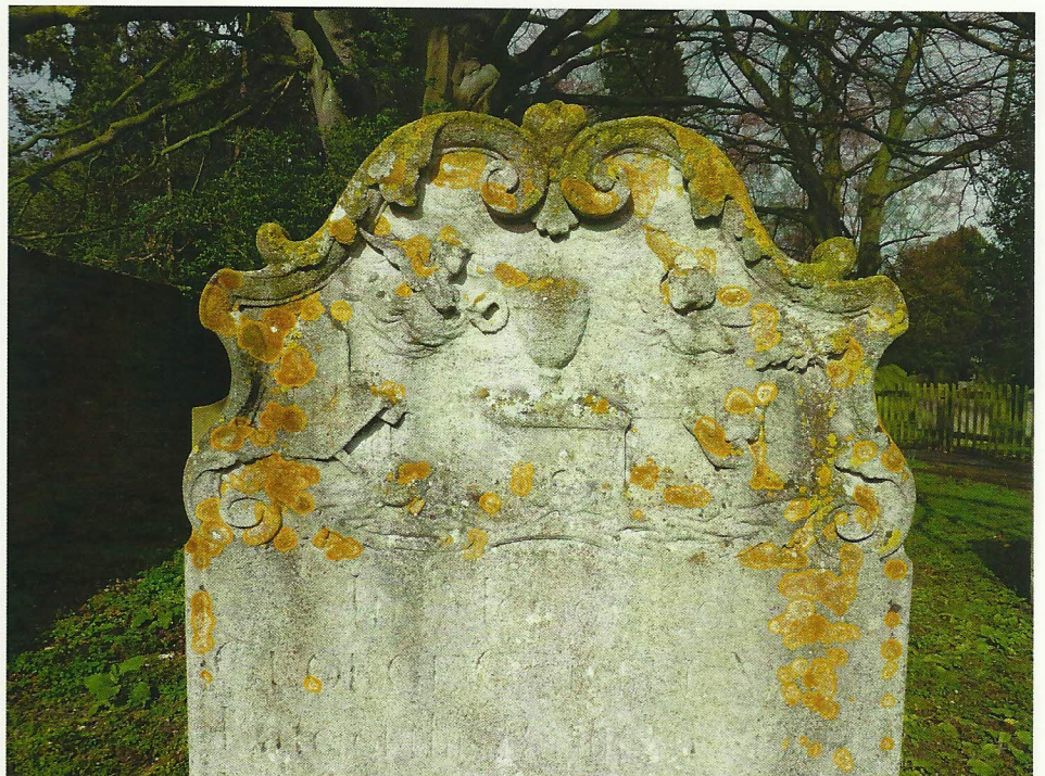
The Carter headstone in 2012. Surface erosion and lichen are compromising the legibility of the relief carving.
