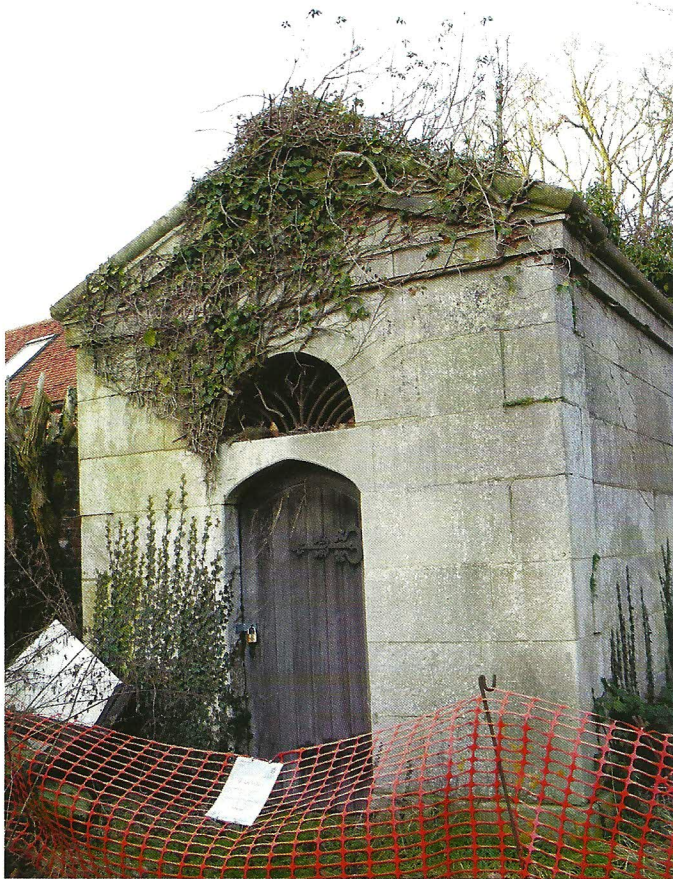
The elegant Lowndes Mausoleum, built in smooth ashlar with relatively few mouldings, before and after restoration.
