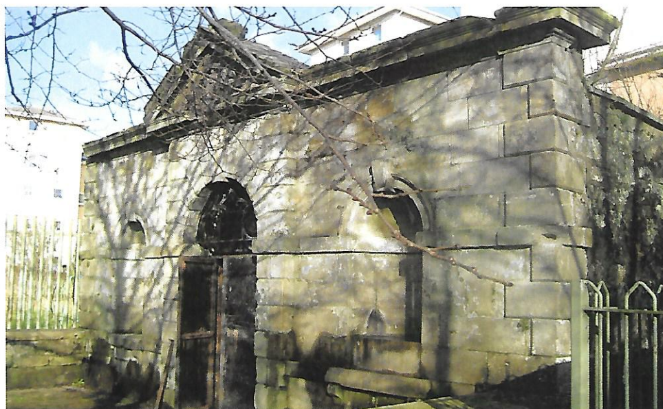
The Wauchope Mausoleum viewed from the South. Image: Historic Scotland
