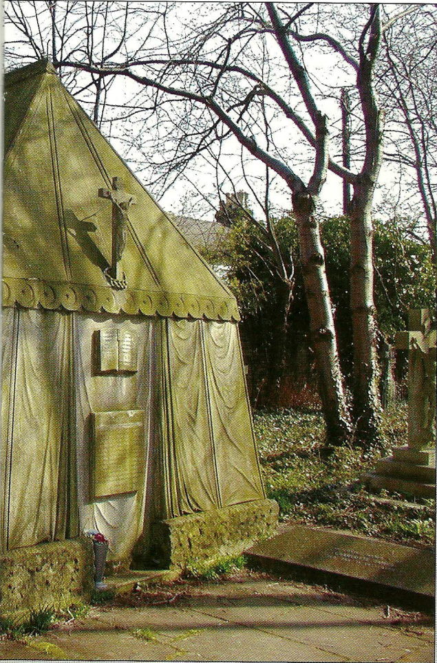
Restoration work began. © Holden Conservation
