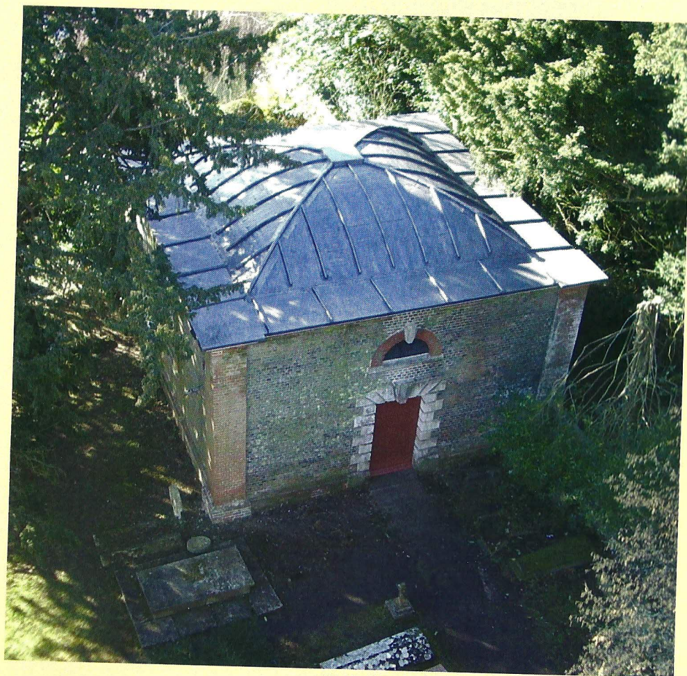
Heathcote mausoleum today following our recent work
